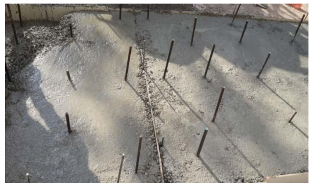
Figure 7 Provision made for Measurement of Temperature at various Intervals
