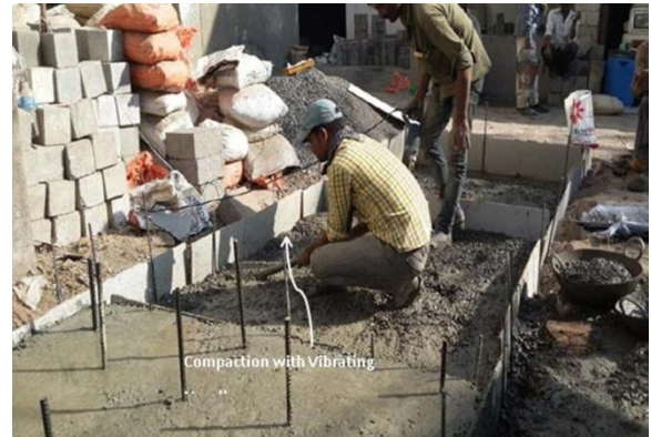
Figure: 6 Compaction with Needle Vibrator and preparation of Base Course
