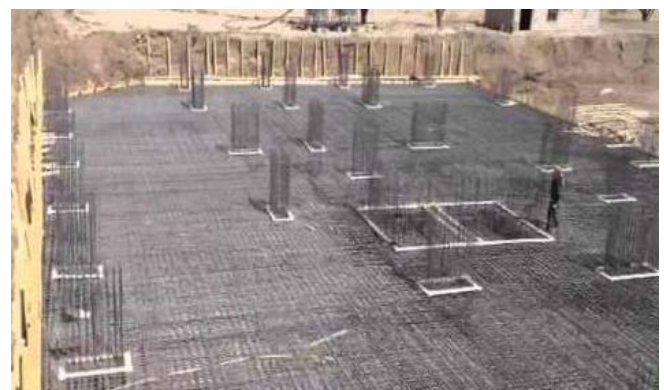
Fig 6: Mat or Raft foundation
