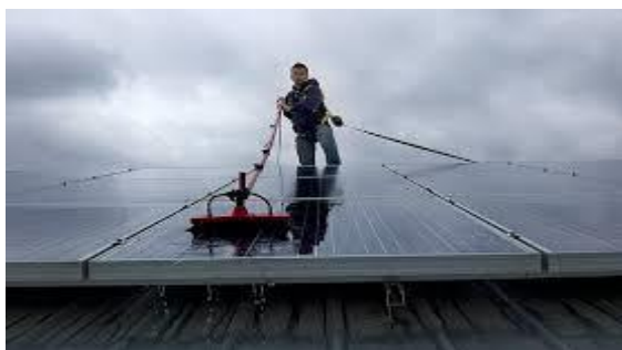
Fig - 5: shows suction cleaning
