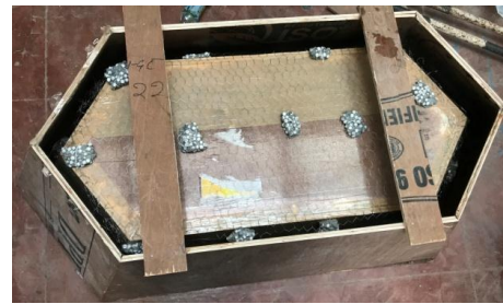
Figure 3. Reinforcement Placing
