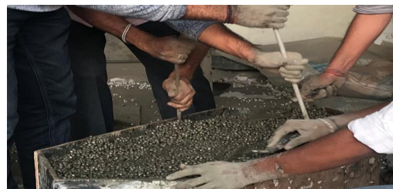
Figure 4. Showing Placing and Compaction of Concrete
