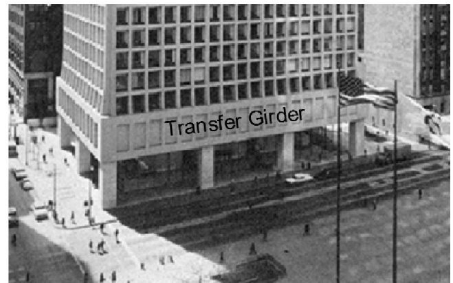
Fig -1. Transfer girder
