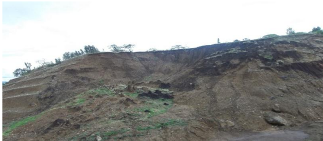
Figure 2.1: portion of embankment project site
