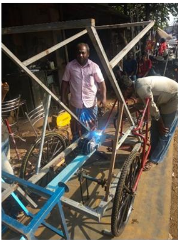
Fig -9: Implementation Works
