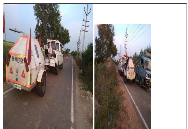
Figure 5: Few snaps taken during FWD Survey
