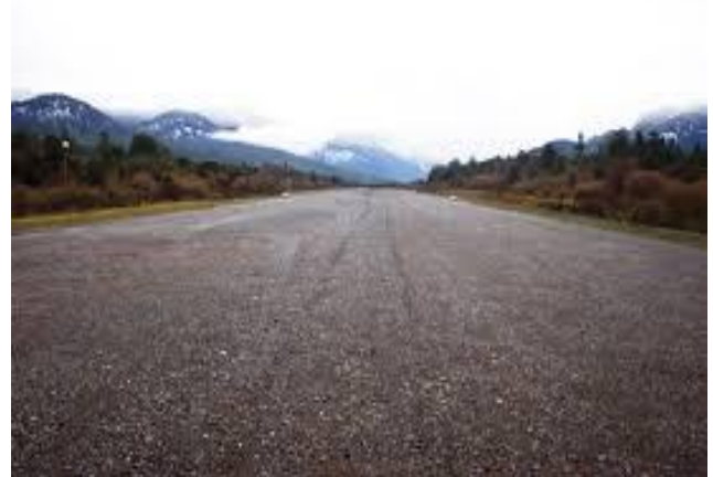
Slag used in sub grade
