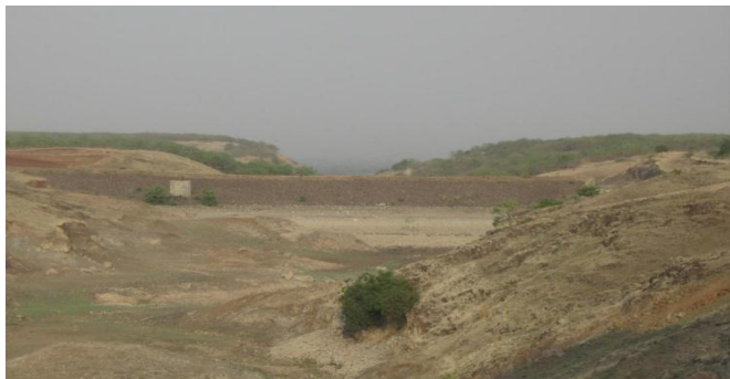
Fig-6-Progress of work on Site for-Percolation tank
