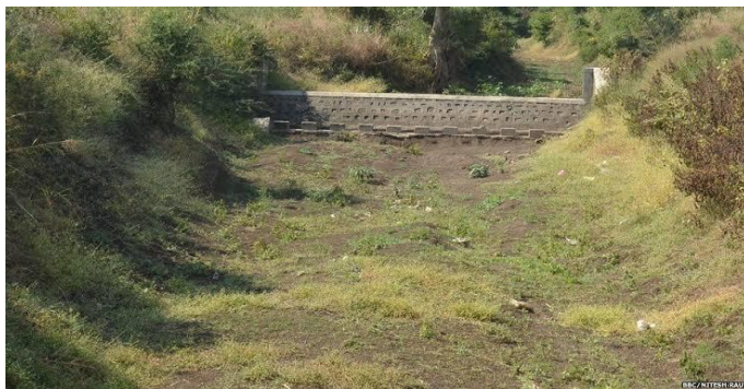
Fig-7-Under repairing of check dam situated on nala of Bhatangali watershed
