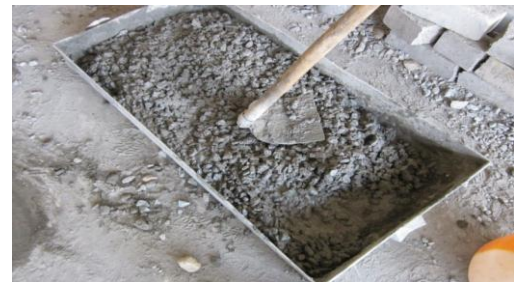
Figure 3. Wet mix of concrete
