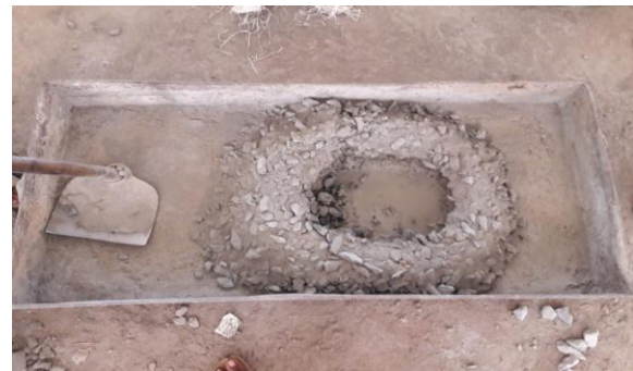
Figure 2. Dry mix of concrete
