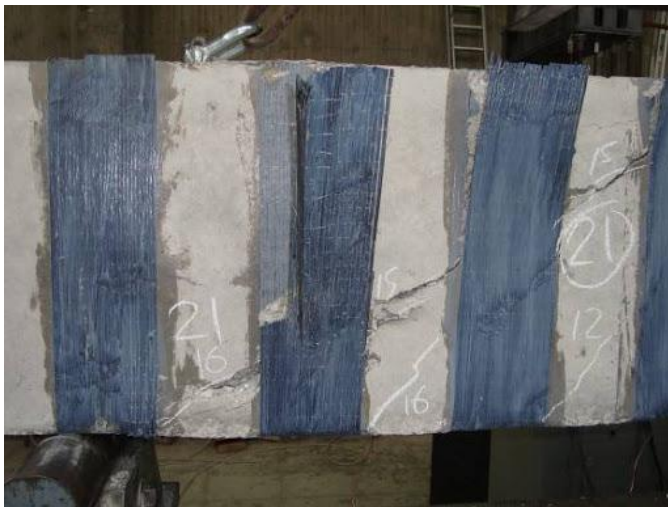
Fig - 4 : Debonding Failure in RCC Beam
