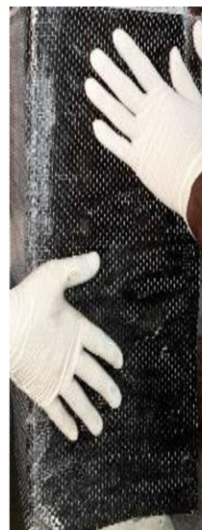
(iv) Wrapping of FRP fabric (v) Rolling to remove air bubbles
