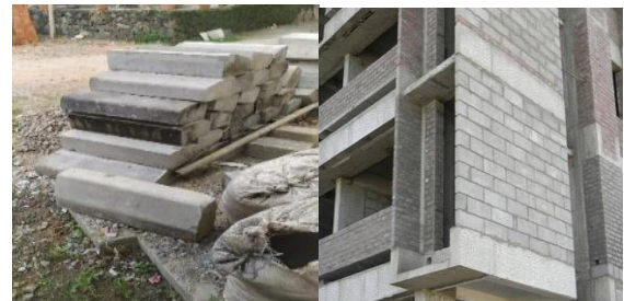
Fig 3 curb casting & partition walls
