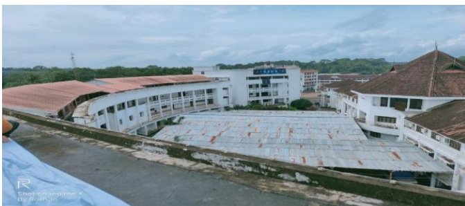
Fig 5. Roof top view (saintgits campus)
