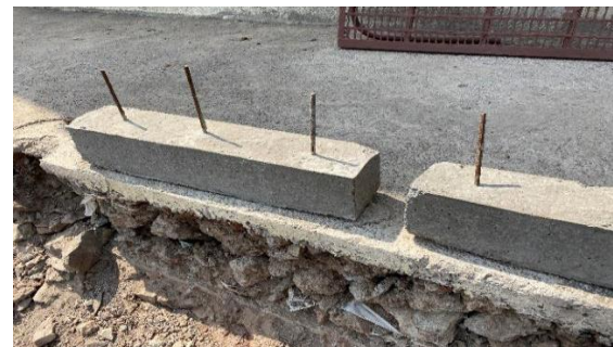
Fig 2- Casting of Beam
