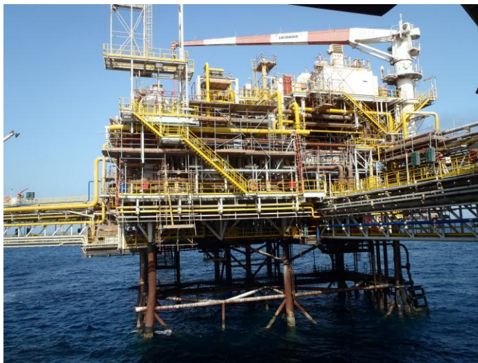
Fig.1. Offshore platform with topside piping (yellow color)
