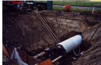
Fig - 2: Pipe Jacking Method
