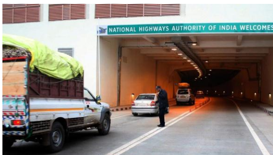
Fig - 9: Chenani-Nashri tunnel, India's longest highway tunnel on the Jammu-Srinagar national highway.
