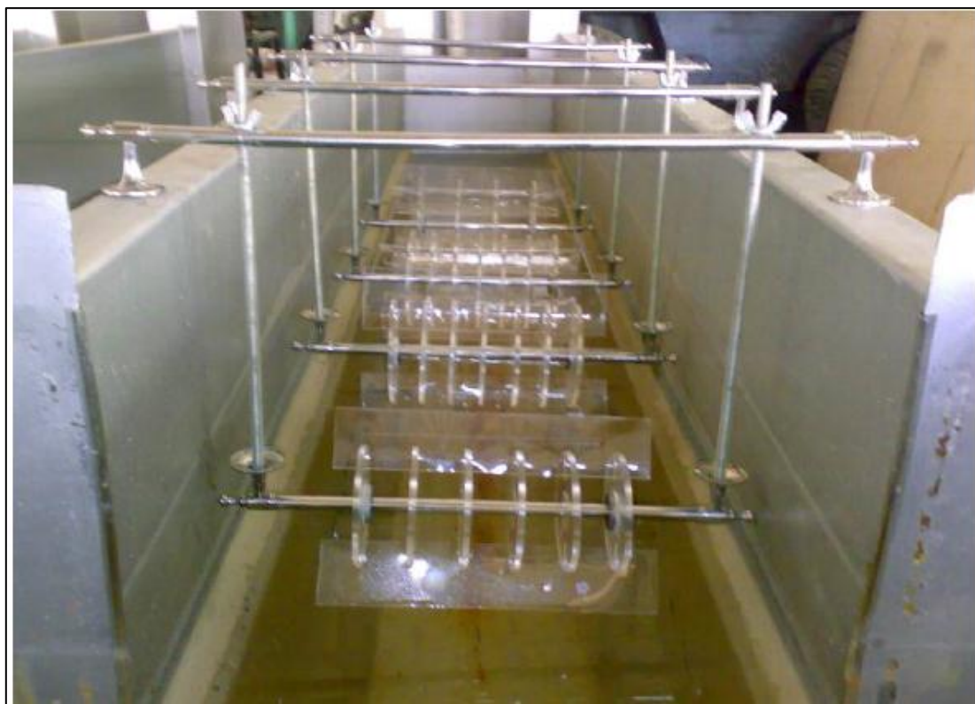
Installation of self -RBC discs on the channel
