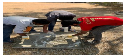
Fig 3.8.10 Concrete Preparation
