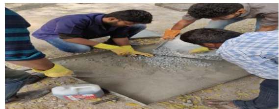
Fig 3.8.9 Mixing of concrete
