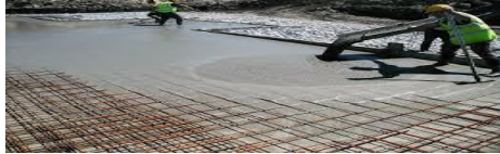
Fig1.1 Placing of Self Compacting Concrete
