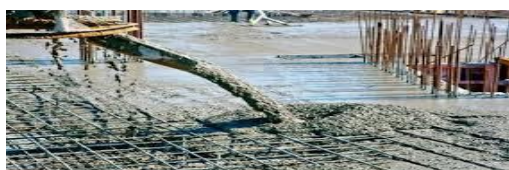
Fig1.2 Application of Self Compacting Concrete
