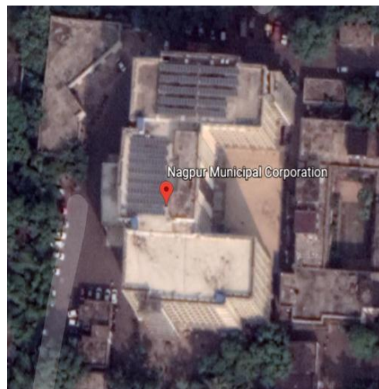
Fig -4: NMC Building
