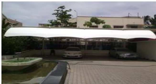
Fig. no.5:- Fibre sheet shed
