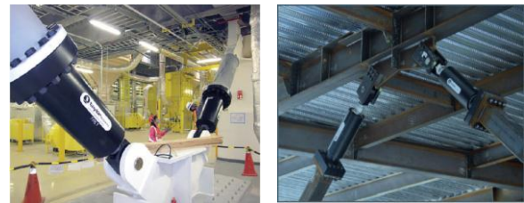
Fig -1: Viscous damper
