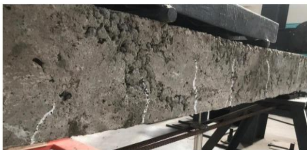
CFS Retrofitted beam Crack pattern
