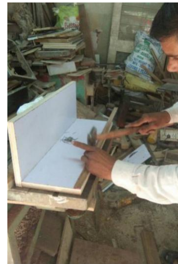
Fig.16 Mould creation using ply wood
