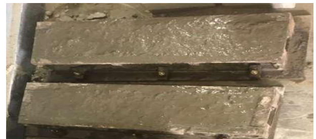
Fig -5: Casting Beams
