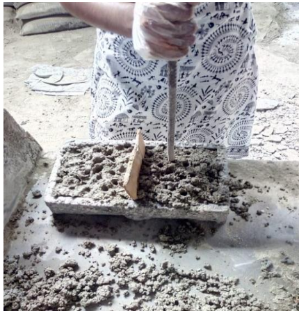
Fig-3: Compacting of Papercrete
