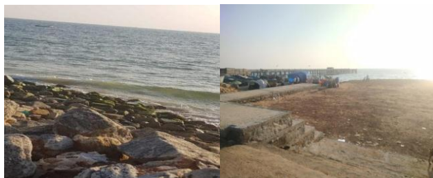
Fig 13 . Present condition of Valiathura
