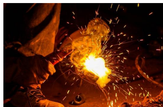
Fig-4.2. Arc Welding
