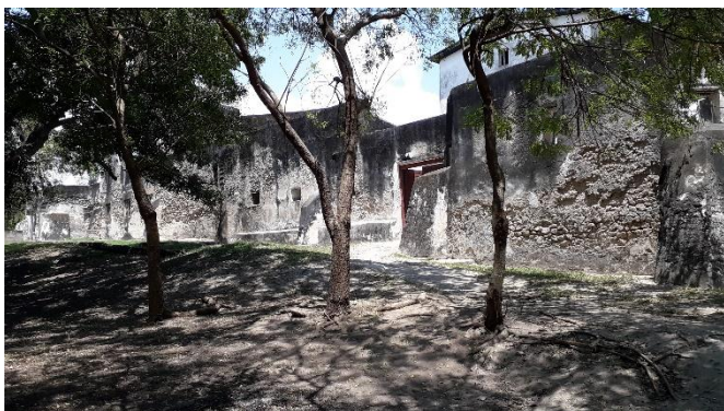
Figure 13: The View of Bagamoyo Old Fort Source: August 2019 Field Survey
