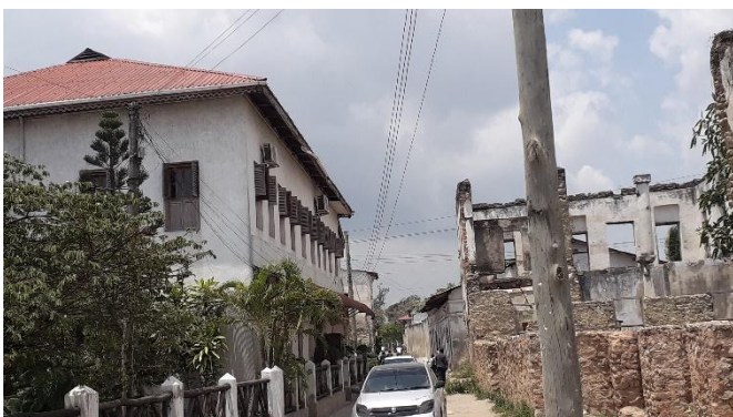
Figure 11: Deterioration of Old Stone Buildings along India Street in Bagamoyo Source: August 2019 Field Survey
