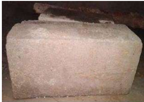
Fig. 5. Demoulding of beam
