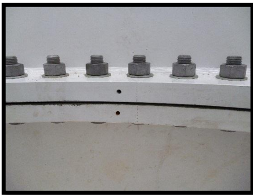
Fig -3.After bolting
