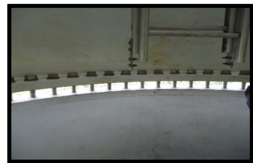
Fig -2. Inserting bolting in tower
