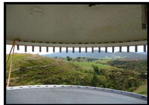
Fig -1. Before Bolting in tower
