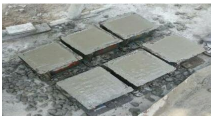
Fig. 3. Moulding of Concrete
