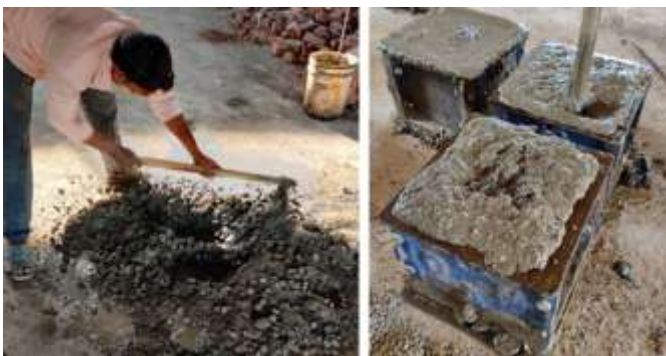
Fig -10: Preparation of concrete and casting
