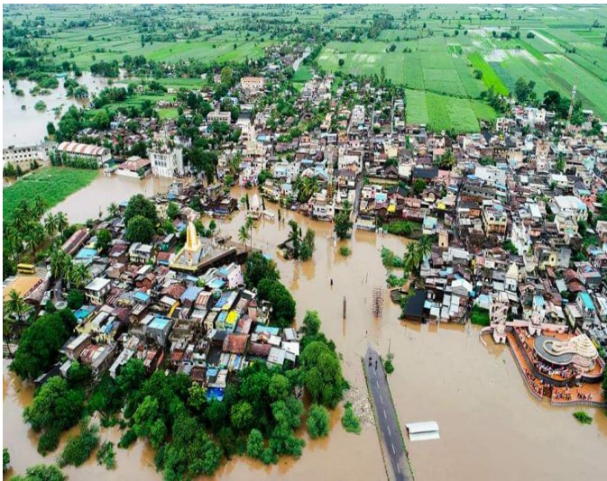
Fig 1.4 Krushna Bridge during Flood
