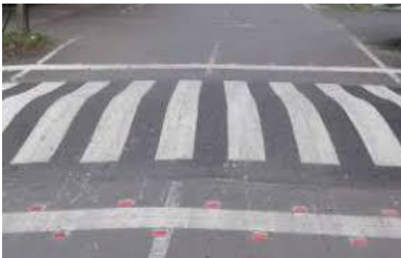
Figure 1. Conventional concrete speed breaker
