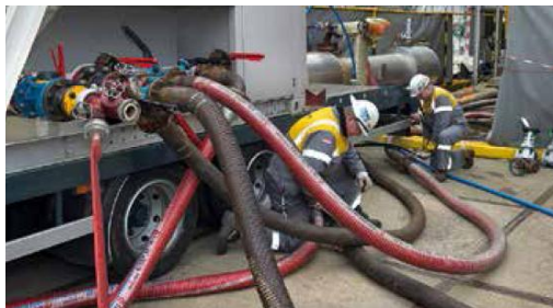
Fig -5 Chemical Cleaning of Columns, Exchangers and Vessels
