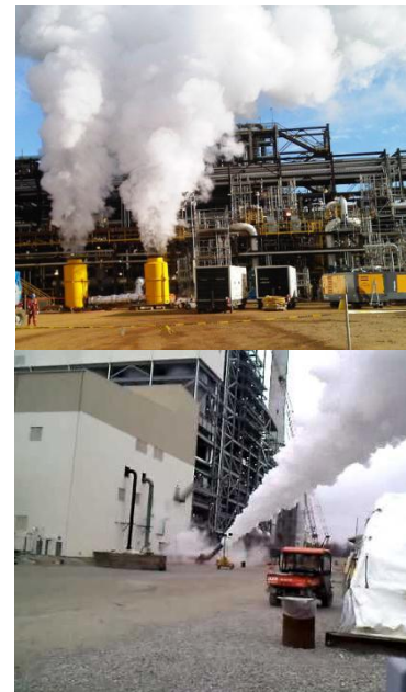
Fig -2: Steam blowing in Process plant
