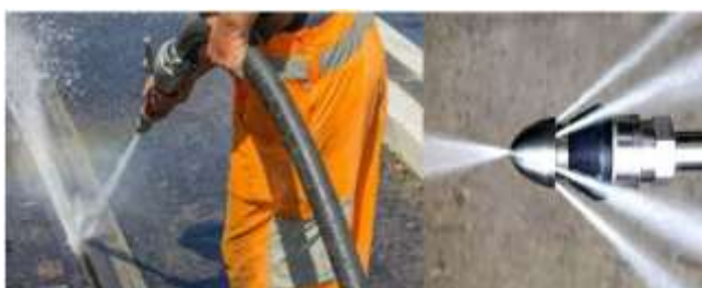
Fig-2 : Hydro Jetting Method
