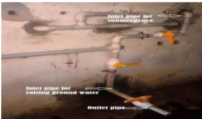
Fig 2: Plumbing arrangement
