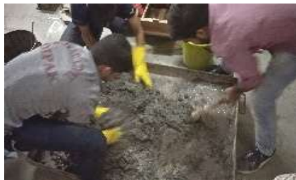
fig no.2 geopolymer work
