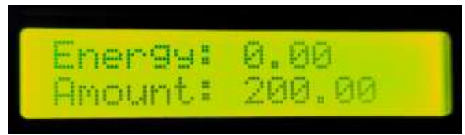
Fig 8: Meter readings before switching ON the load
