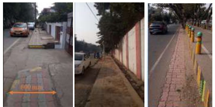
Fig 3: Poor design of the footpaths and their continuity is really challenge to use them
