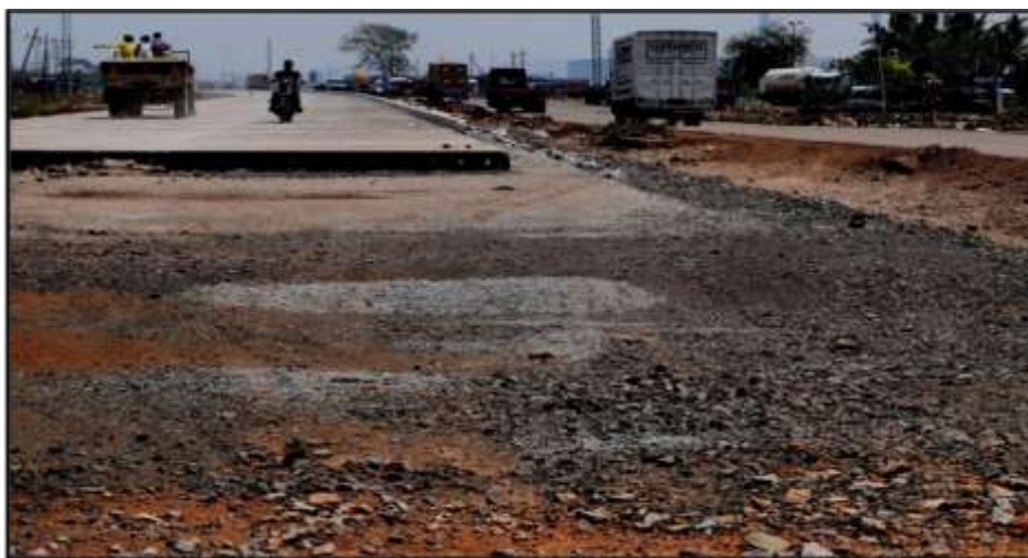
Fig 2. Slag aggregates being used in the construction of pavements
