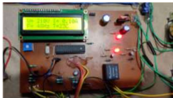
FIGURE 4:- Measuring parameter of transformer on display screen
