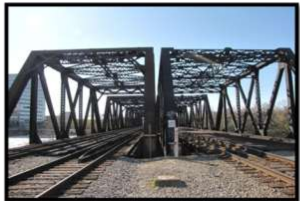
Fig.1 CSX Railroad (CSX) and Conrail (CR)
