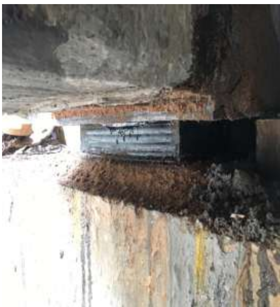
Fig 5. Newly Designed Bearing.
