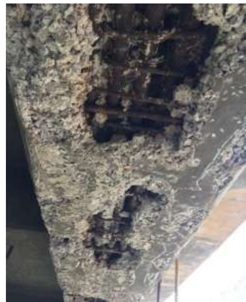
Fig 1. Removing and Redoing of bulb portions of Girder.
