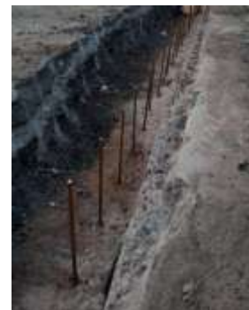
Fig 7. Treatment of Expansion Joints.
