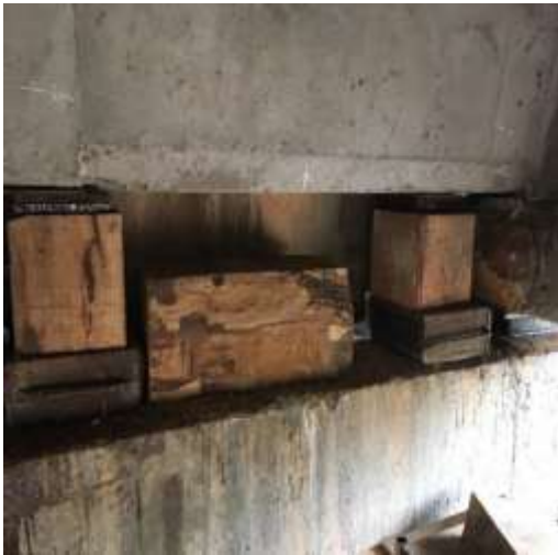
Fig 3. Replacement of Bearing.
