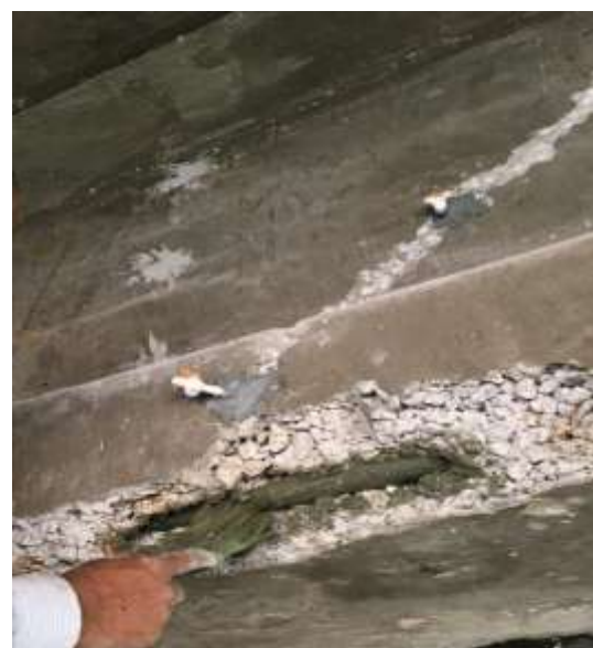
Fig 2. Treatment of Web portions of the Girder.
