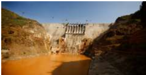
Fig-5: Gibe III hydroelectric power plant dam
