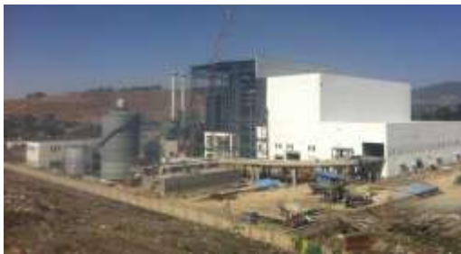
Fig-8: Repie-Koshe biomass power plant
