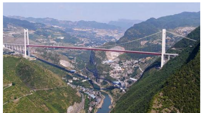
Figure.7: Chishui River Bridge
