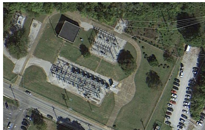
Fig. 2: Aerial view of the instrumented electrical substation.
