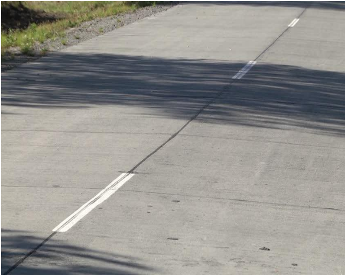
Figure: Concrete Pavement
