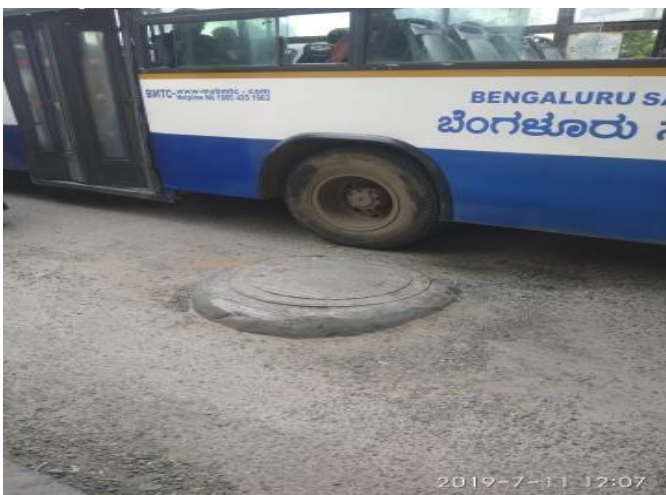
Fig -2: MANHOLE AT THE CENTER OF ROAD AT BLACKSPOT 6
